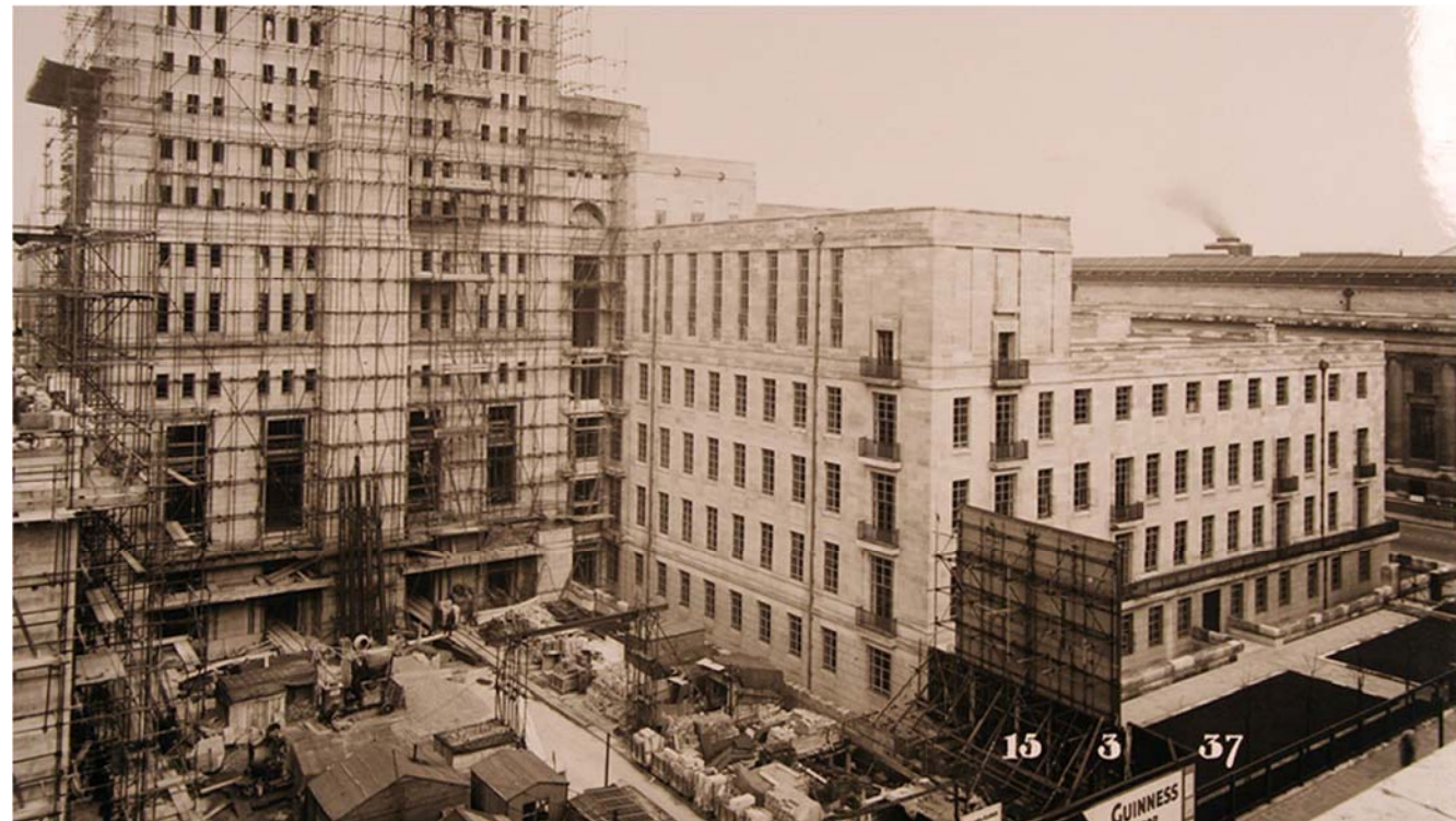
Figure 12 A photo of 1937 showing the construction of the tower of the Senate House. Source: Historic England.
