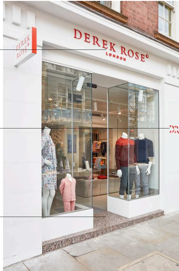
PRECEDENT SHOPFRONT ENTRANCE AT DEREK ROSE STORE, KNIGHTSBRIDGE
