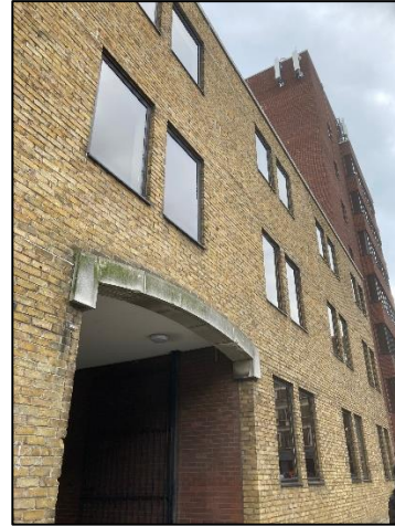
Figure 4: The exterior from Acton Street
