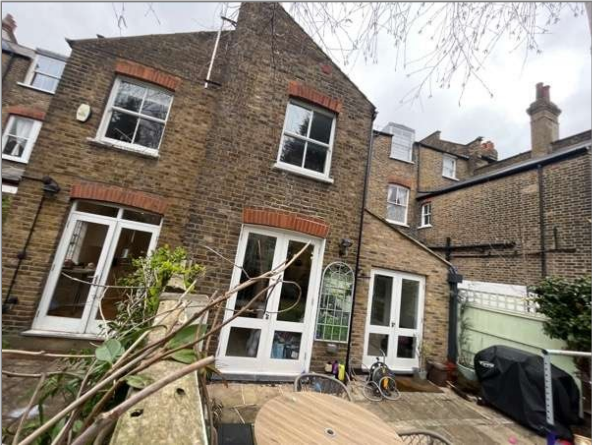
View - Rear Neighbouring Elevation
