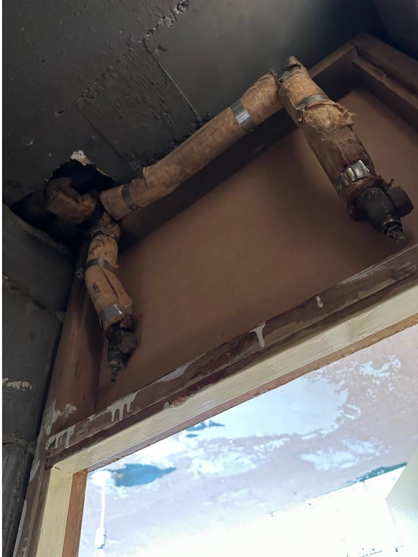
Figure 7: Obsolete pipework in kitchen cabinetry to be removed.
