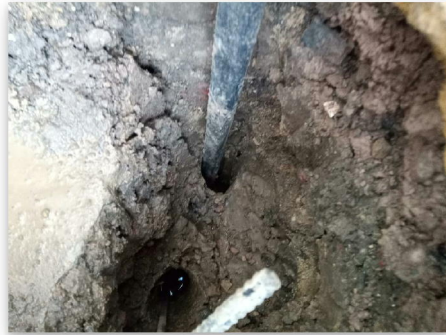
Fig 1.2: Trial Hole 1 Footing
