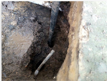
Fig 1.3: Trial Hole 1b Footing
