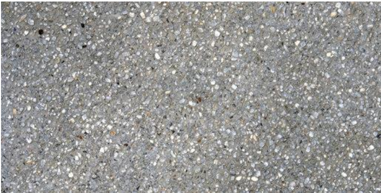
Pic 1: Exposed aggregate concrete
