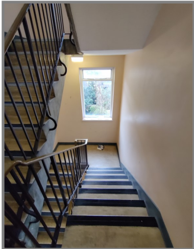
1. Communal stairwell, providing access to the 2nd floor flat
