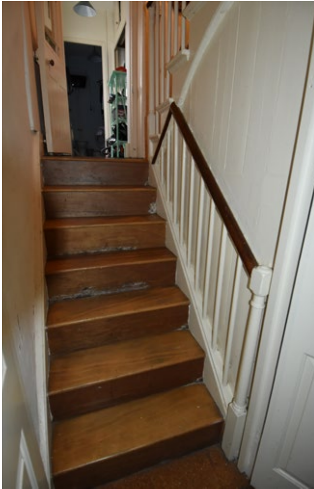
3.12 Staircase flight from lower ground floor to the half landing. The treads have been rebuilt (2023, Donald Insall)
