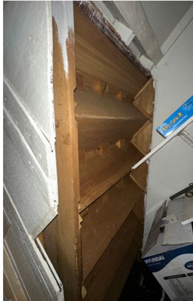
3.13 The underside of the lower ground floor stair in LG5, showing its modern construction (2023, Donald Insall)
