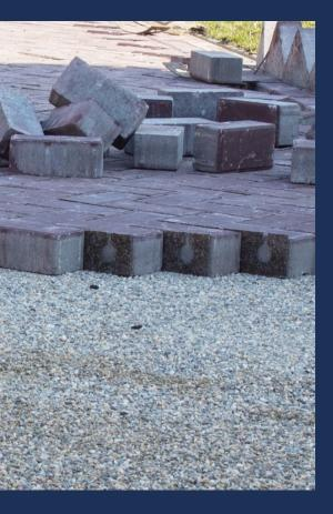
Drainjoint permeable paving is easy to install and can be used with many different materials. Removing the need for pavers to carry nibs or extensions and avoiding the requirement for large, unsightly aggregate joints, the system preserves the beauty of the paving material.
