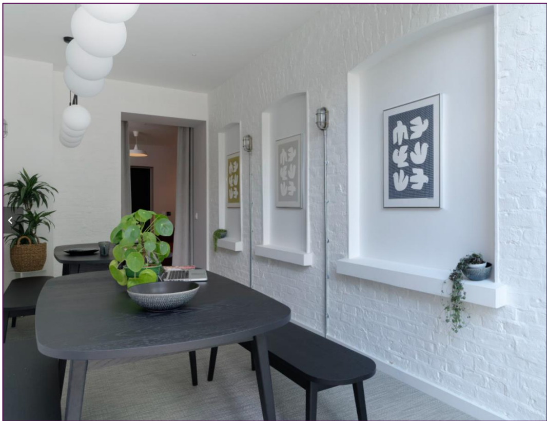
Figure 1: Existing blocked-up internal windows
