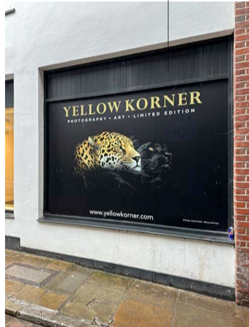
EXISTING TIMBER PANELLED CLAD FASCIA
