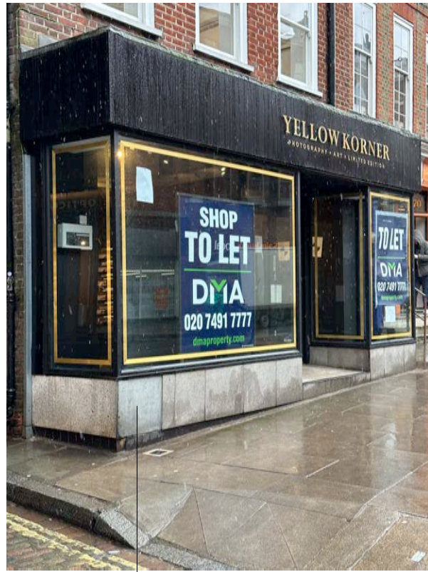
EXISTING MIS-MATCHING & DAMAGED STONE TILED STALL RISER CLADDING
