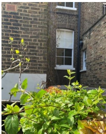
Figure 03 – Ground floor rear window
