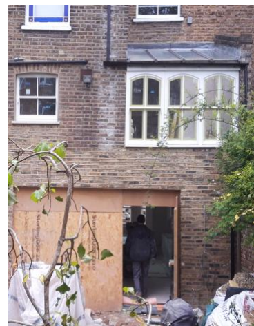
11 Laurier Rd rear extension
