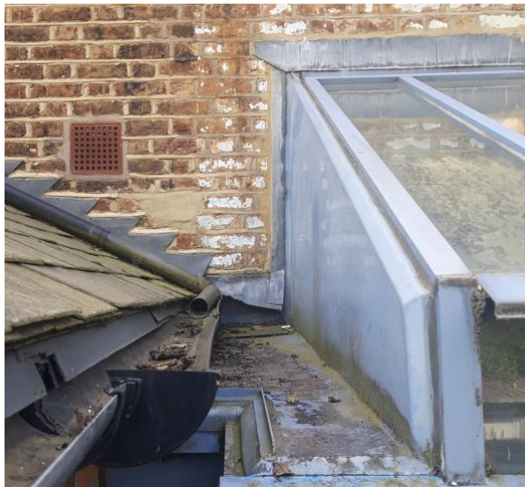
Existing junction and gutter.
