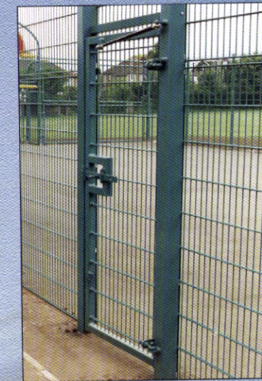
1m wide, single leaf gate with self-closing mechanism & over panel
