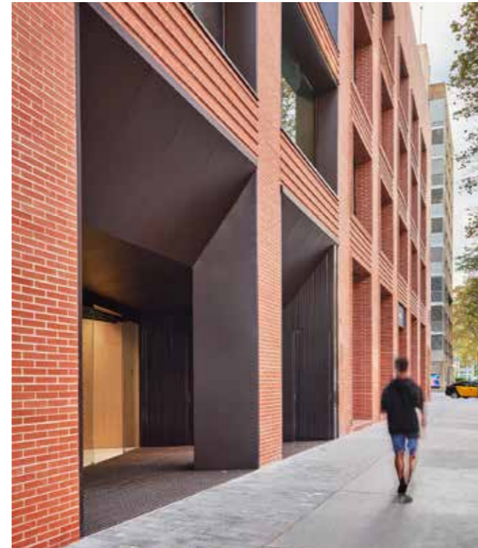
Example metal facade
