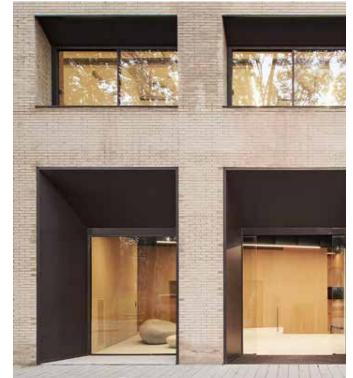
Example metal facade
