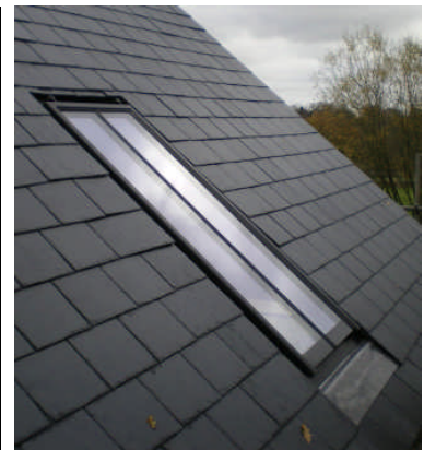
Image 2. Conservation rooflights for a slate roof example Installation guide provided
