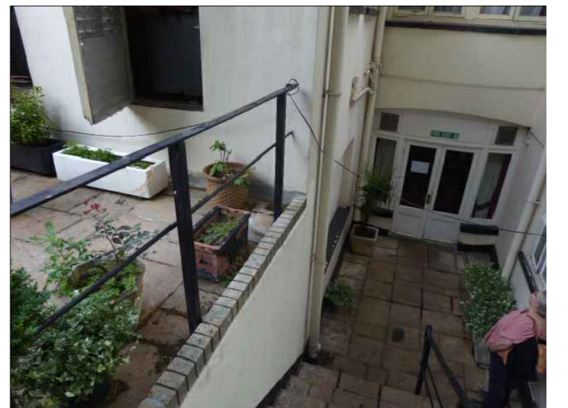
Existing Lightwell 11 Railings
