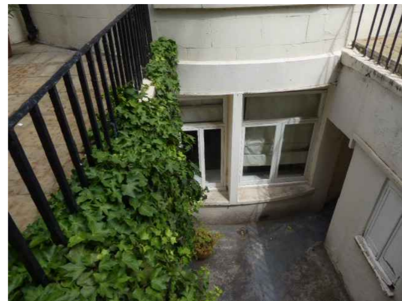
Existing Lightwell 09 Railings
