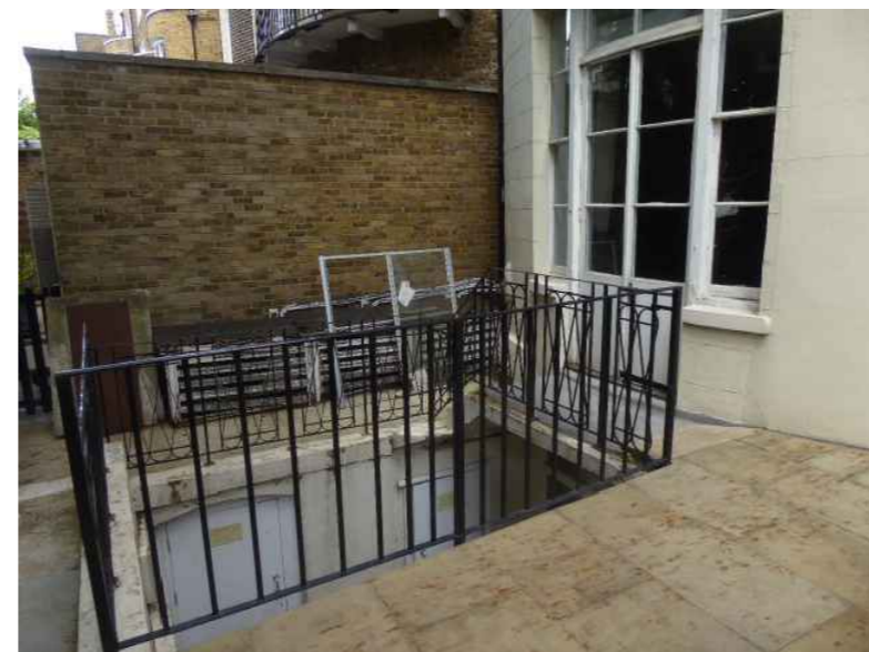
Existing Lightwell 10 Railings
