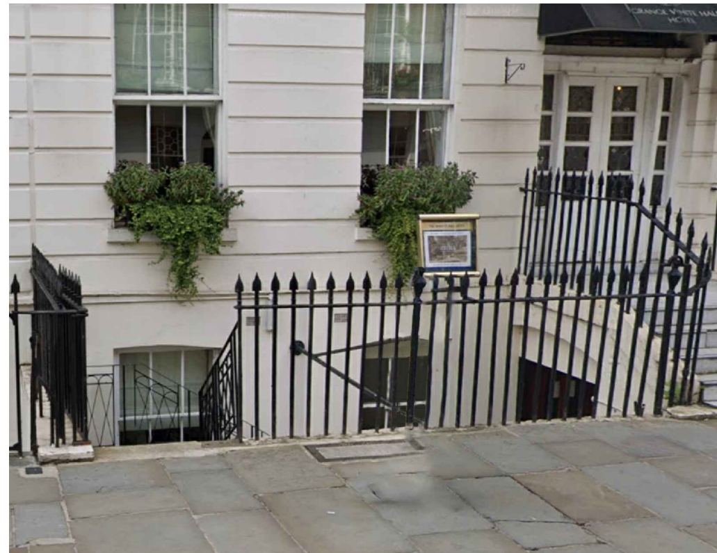
Photograph - Existing external staircase from street level
