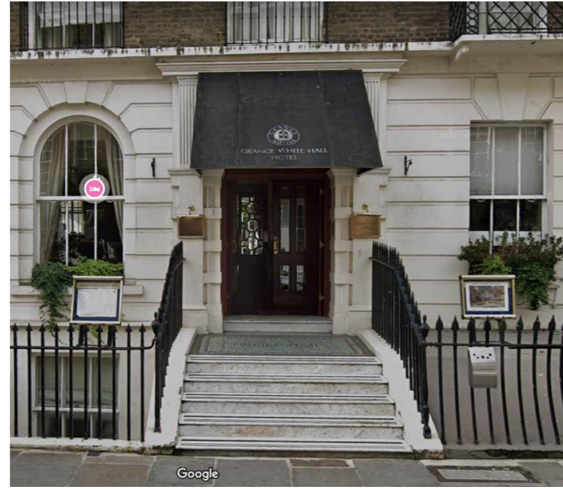
Building No.03 Front Steps with non-original mosaic
