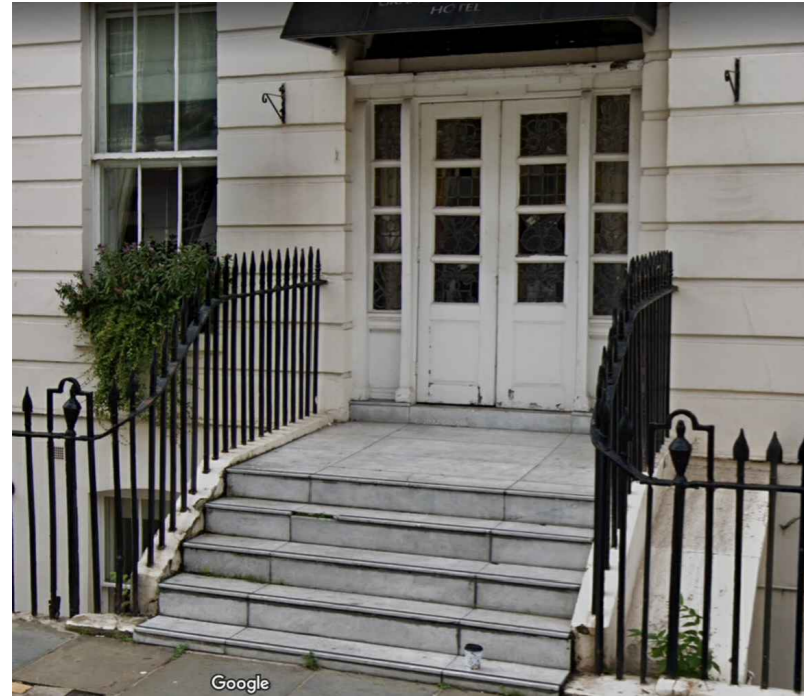
Building No.02 Front Steps
