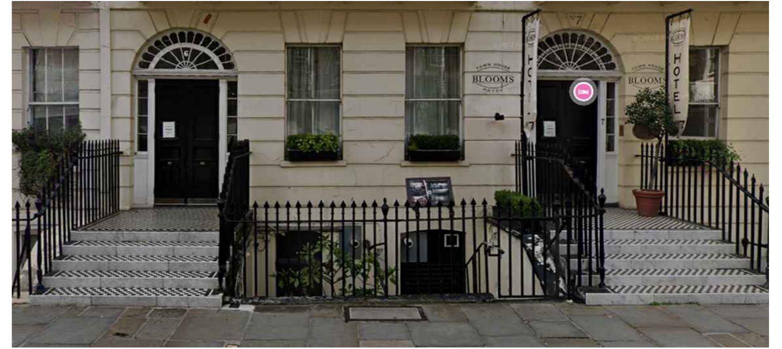
Buildings No.05-06 Front Steps
