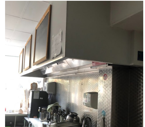
EXISTING OVERHEAD EXTRACTION SYSTEM
