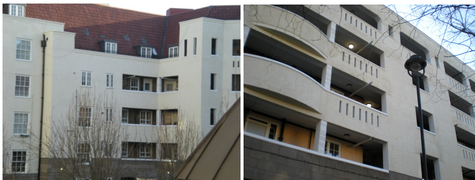
Straight white boiler flues to other flats at Levita House
