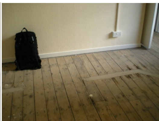
Former partition marking in floor
