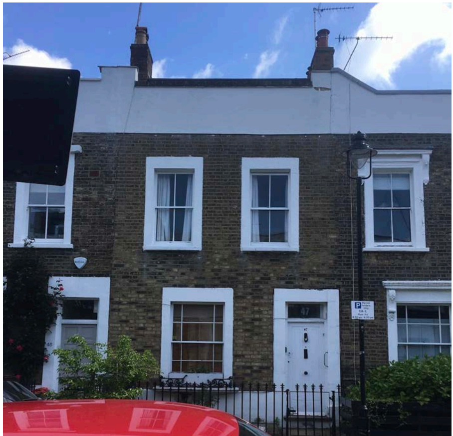
View of 2nd floor extension from pavement directly opposite No. 47 Alma Street
