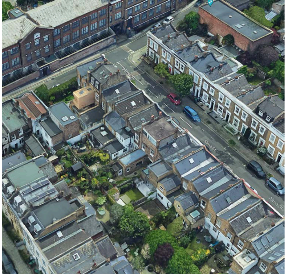
No.s 52 & 41 Alma Street, rear elevation to terrace
