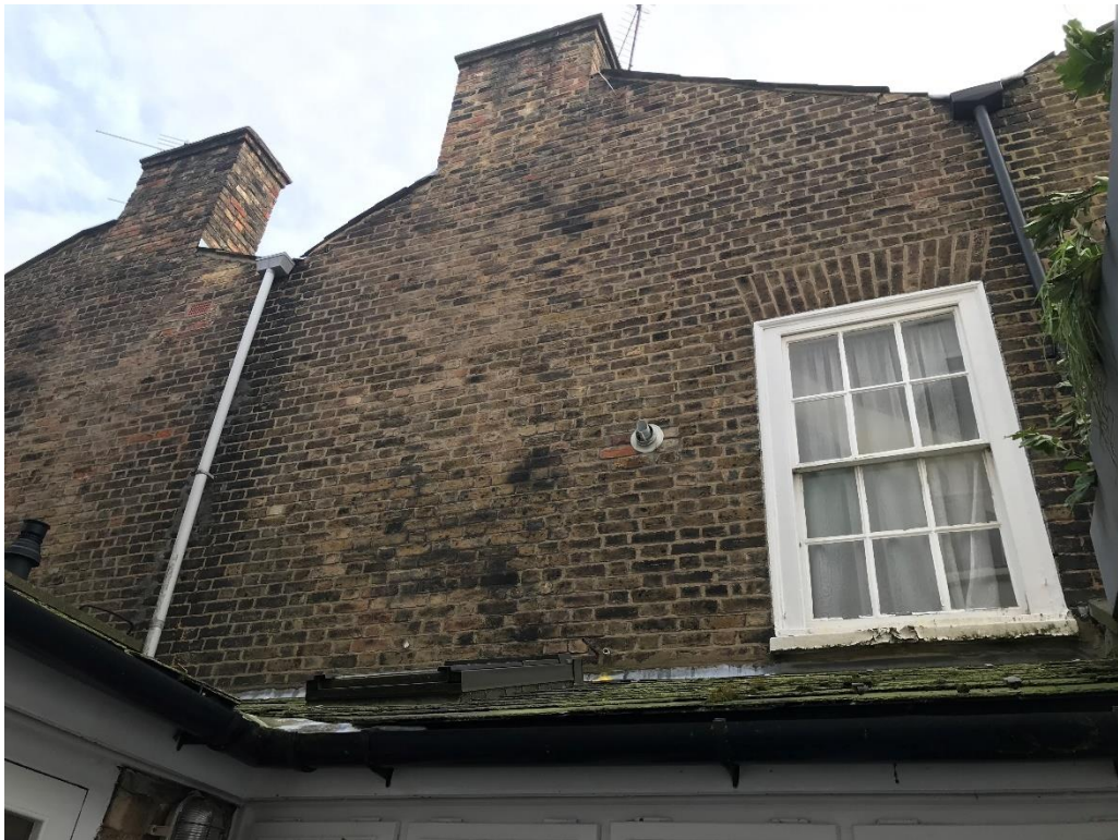
Figure 31: View of rear elevation
