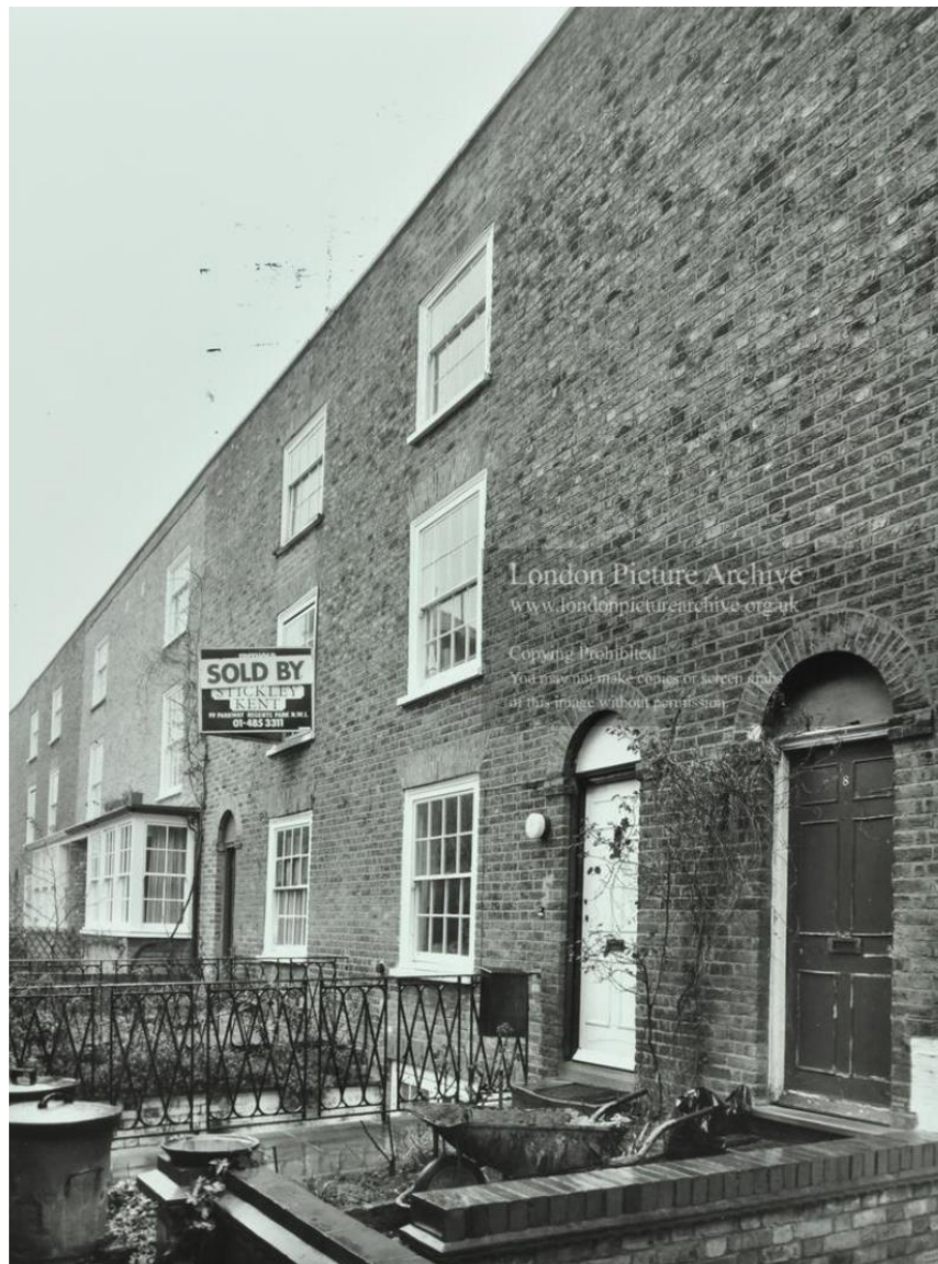
Figure 16: View of Benham's Place from the east photographed in 1975 with Nos. 4-5 rebuilt.
