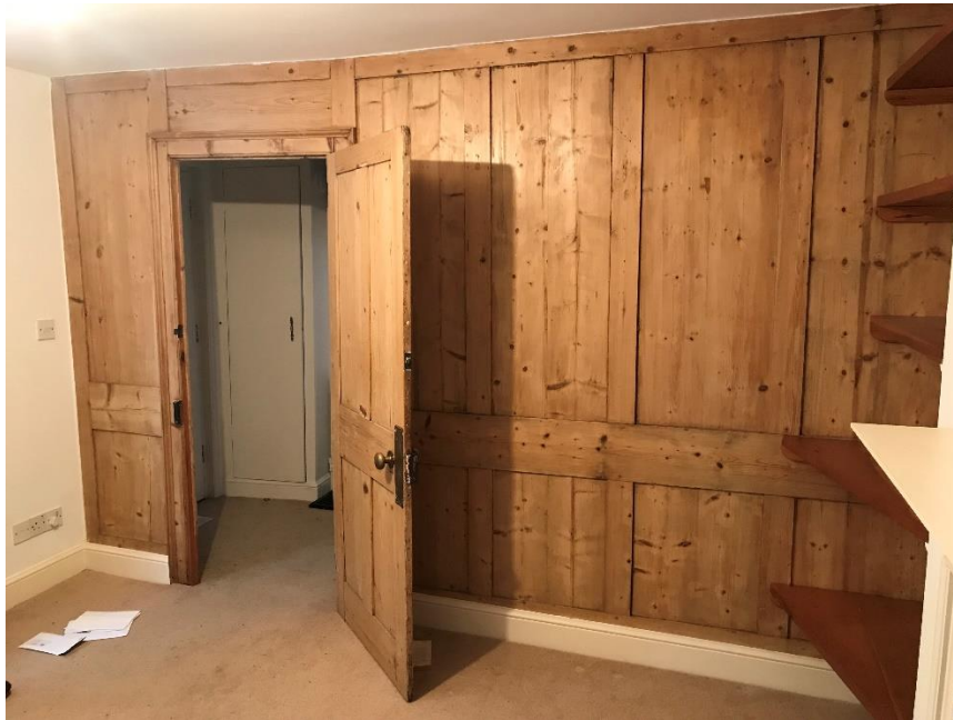
Figure 21: Timber panelled partition to the ground floor living room.
