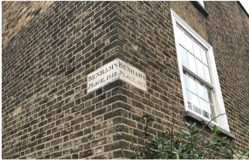
Figure 17: Street name carved into stone quoin to No. 1 Benham's Place
