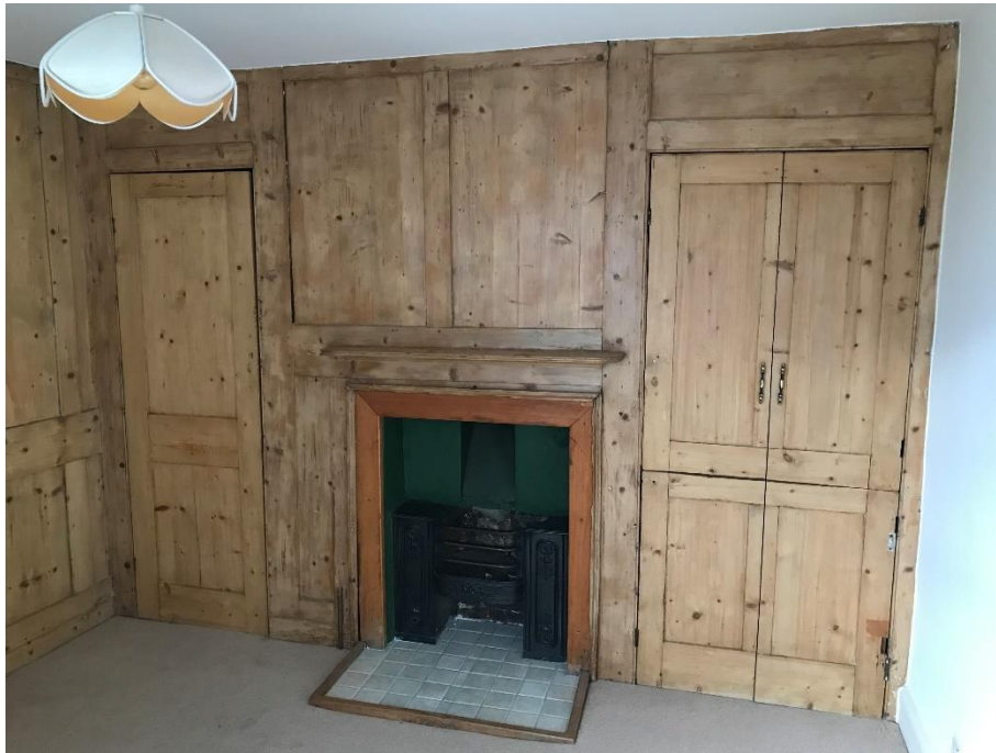
Figure 23: Fireplace and panelling to first floor room
