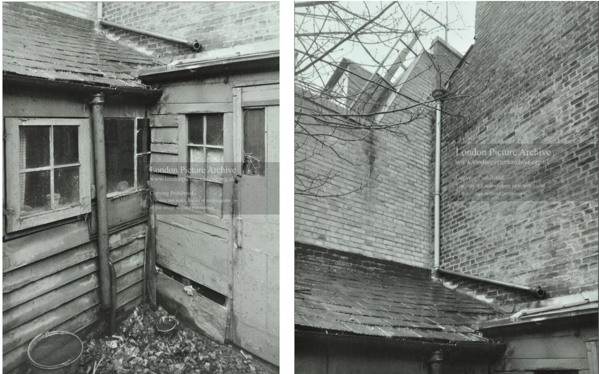
Figure 26: Configuration of original lean-to and outrigger range at No. 6 photographed in 1975. Source: © London Picture Archive
