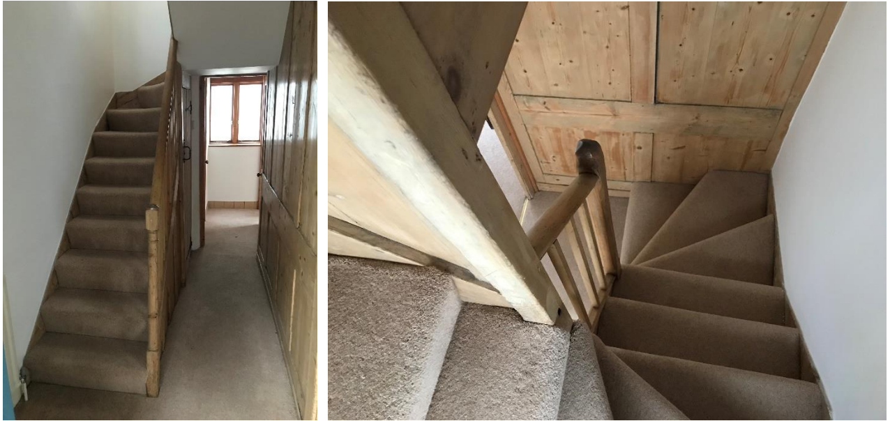
Figure 19: View of entrance / stair hall at No. 2 with timber panelled partition to right (left) and winder staircase between first and second floors (right)
