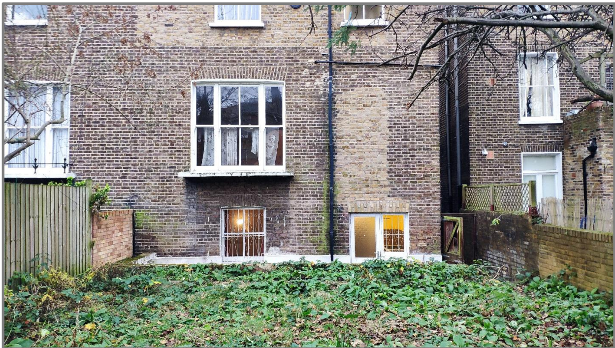
Fig. 6: Existing Rear Elevation - partially subterranean, as the garden level, sits higher to the rear
