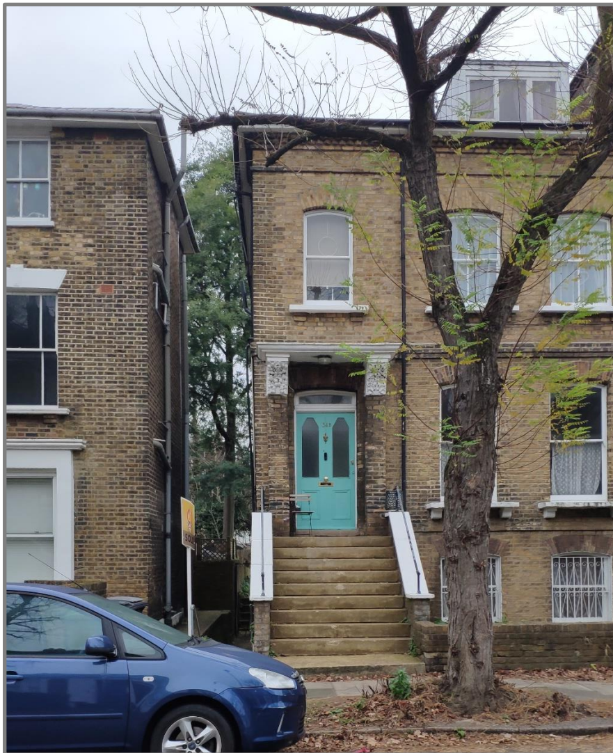
Fig. 1: Existing View - Front elevation 34 Bartholomew Road, London, NW5 2AJ
