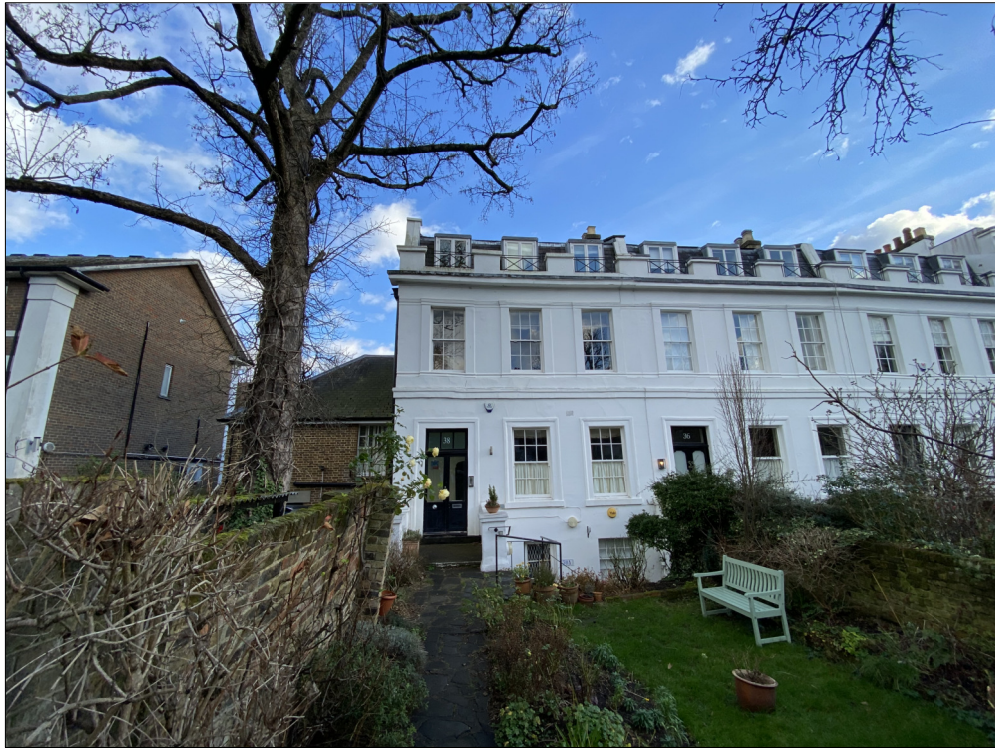
Existing View of Front Elevation
