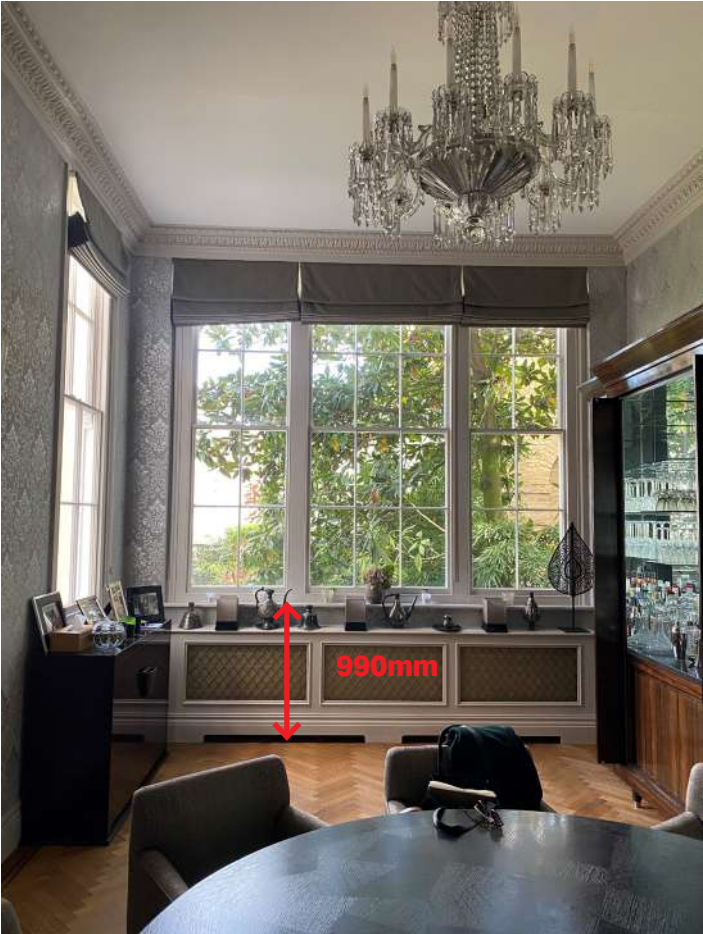
Internal view of dining room window with 990mm cill height as installed during the Donald Insall works
