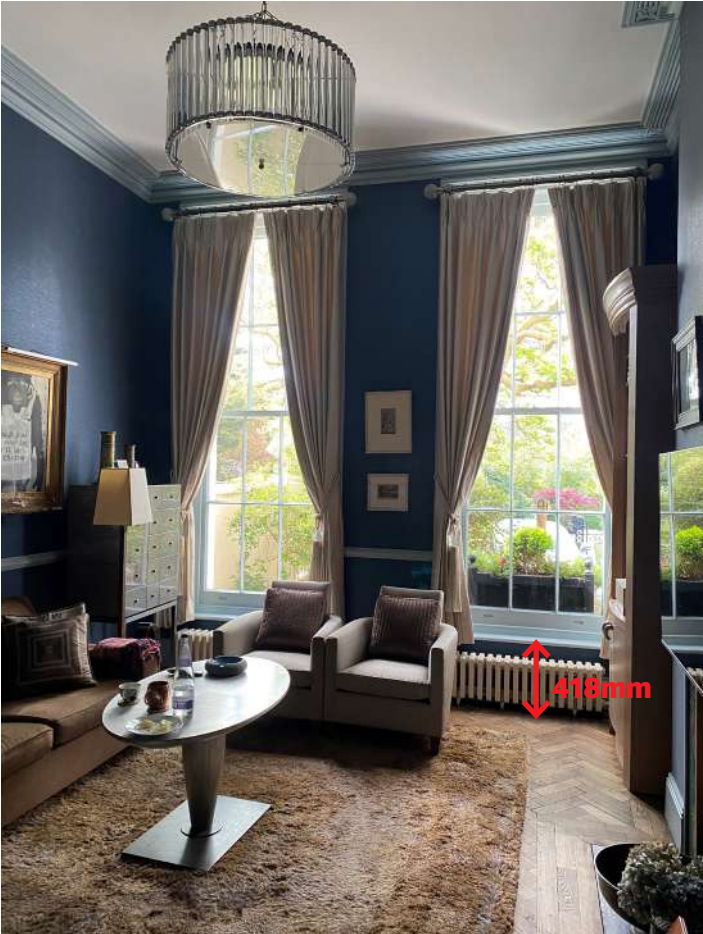
Internal view of study windows with 418mm cill heights of the Papworth extension
