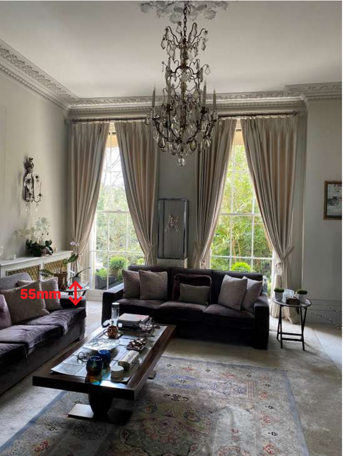
Internal view of original living room windows with 55mm cill heights
