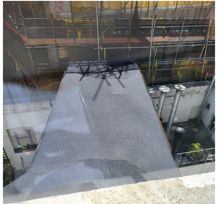
12. Existing extension (Roof)
