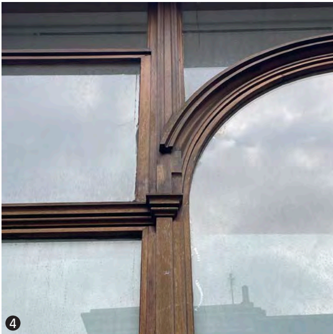
4 Timber mouldings on windows
