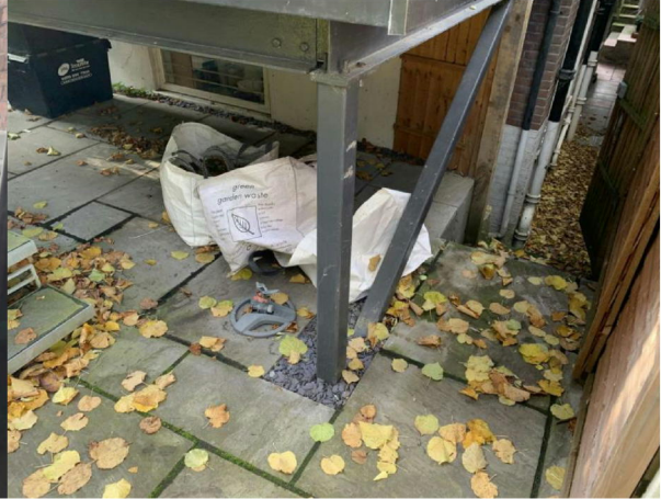
Steel supports, reportedly on pad footings 2.5m-3m deep
