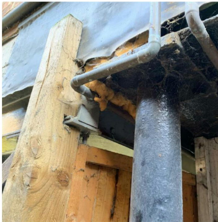
Supporting columns to original projection
