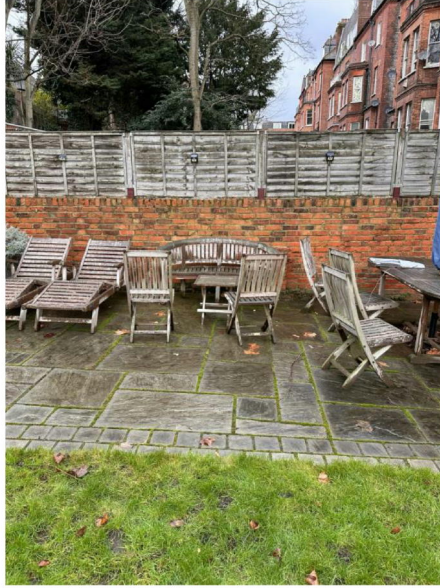
Walling and paving to be removed to facilitate works
