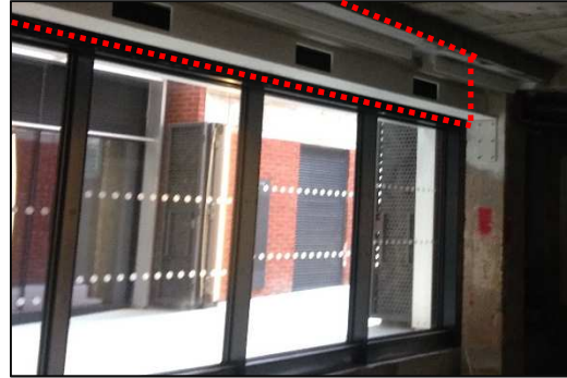
Figure 4.2. Internal photograph of the South glazed façade's lintel
