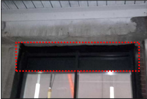
Figure 4.1. Internal photograph of the North glazed façade's lintel
