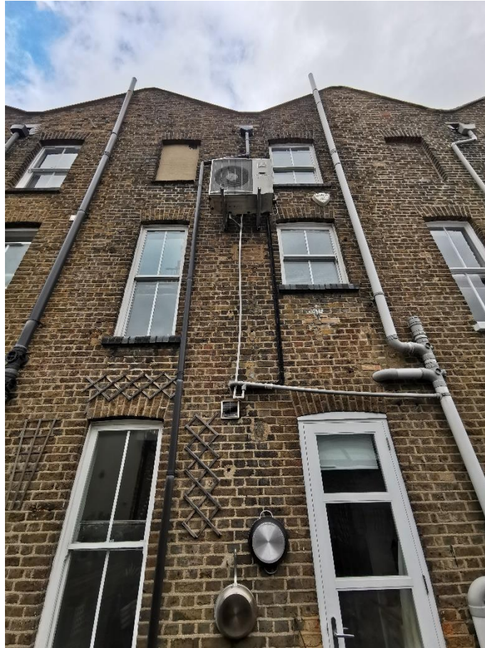
Figure 2 existing rear of the property
