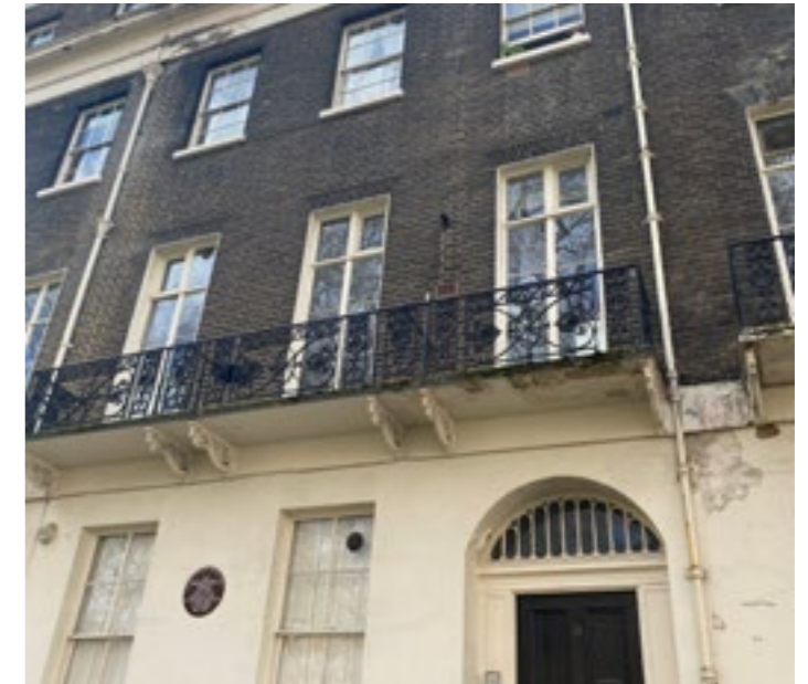
Figure 5.2 Main Entrance services
