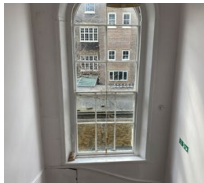
Figure 5.14 Second Floor Stair Window
