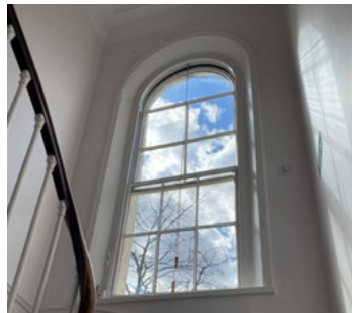
Figure 4.8 Main Stair arched window
