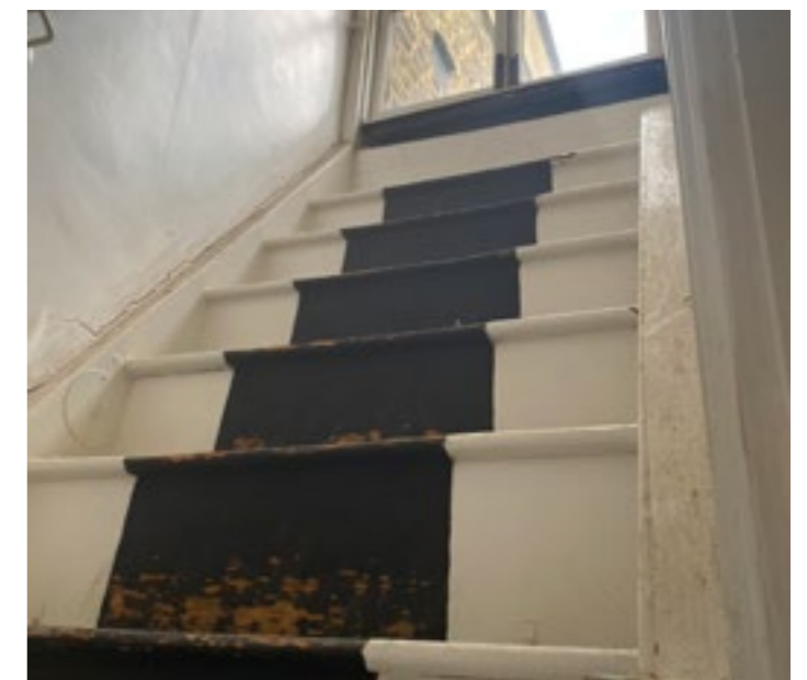
Figure 5.21 third floor roof stair
