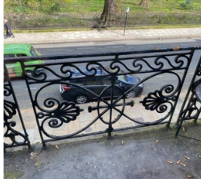
Figure 4.5 Iron Work Balustrade at First Floor
