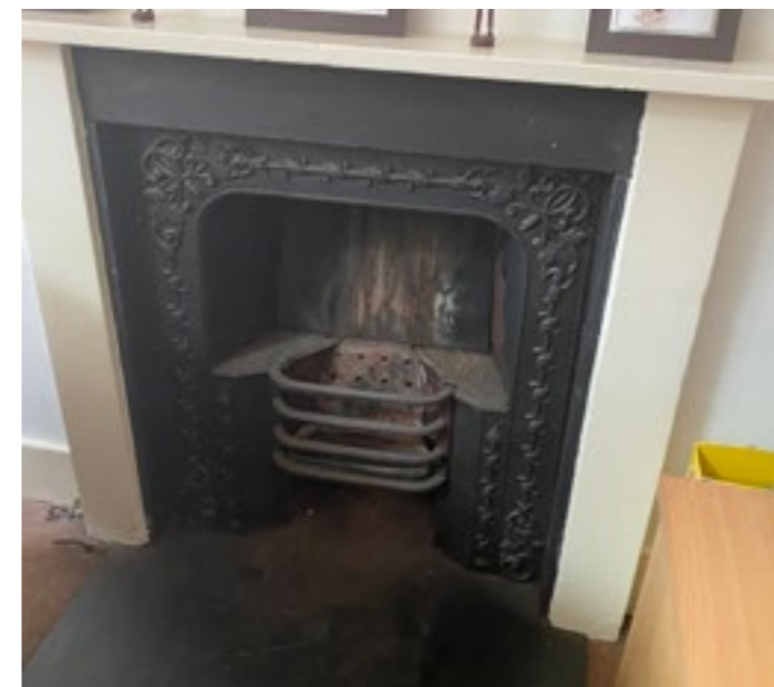
Figure 5.20 Third floor fireplace
