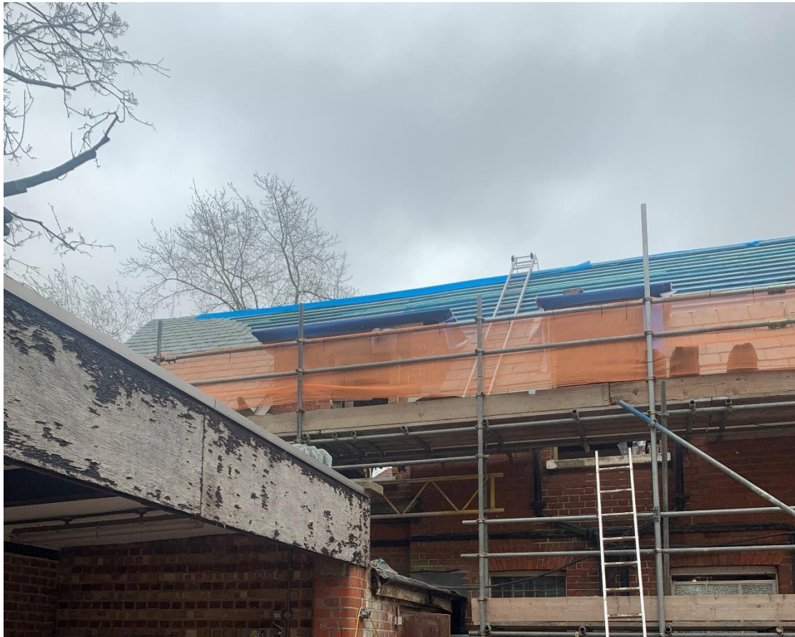
Figure 2: photo from site visit showing the stables being re roofed
