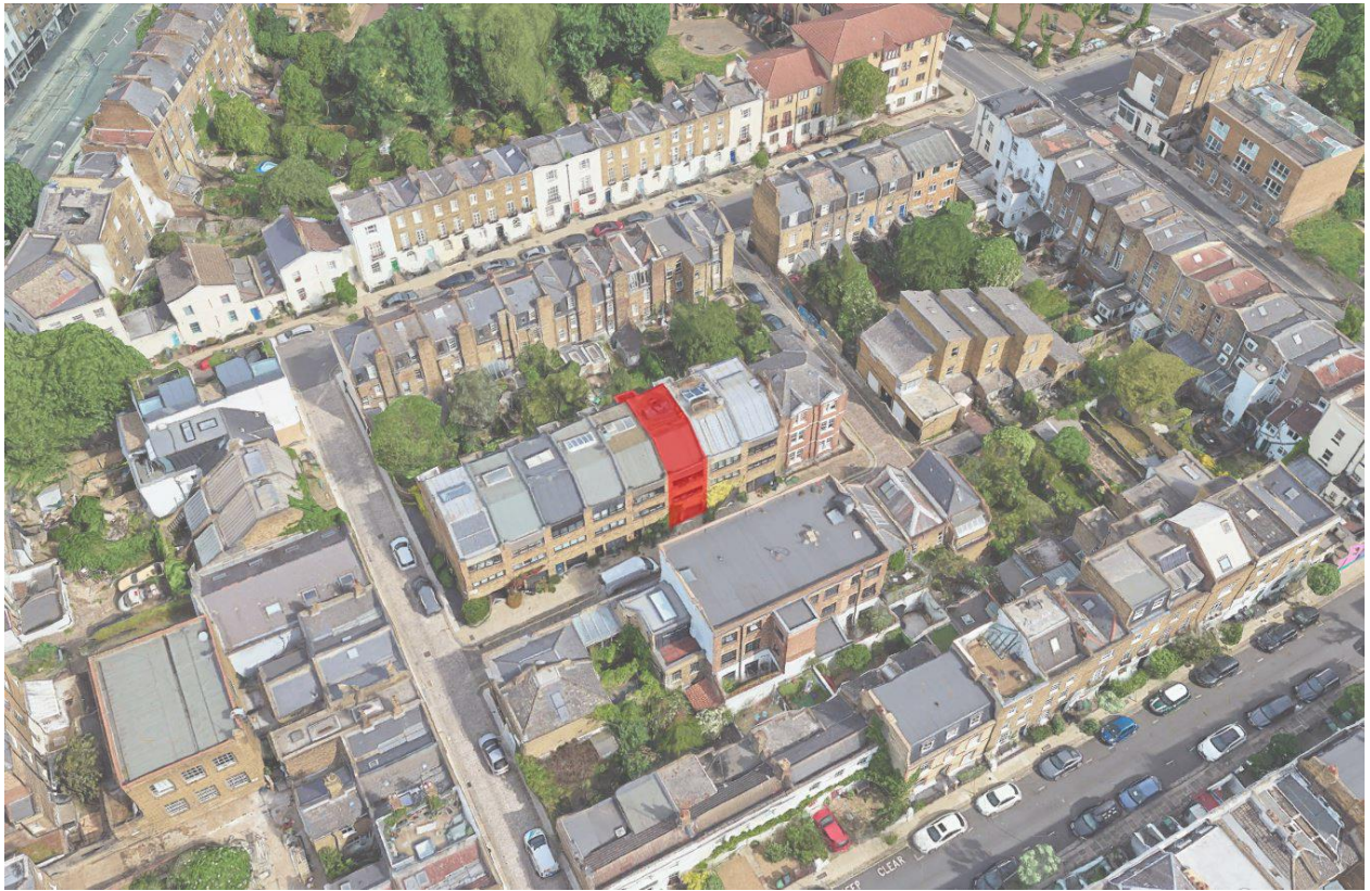
Fig 3. Aerial view showing 17 Jeffreys Place highlighted in red
