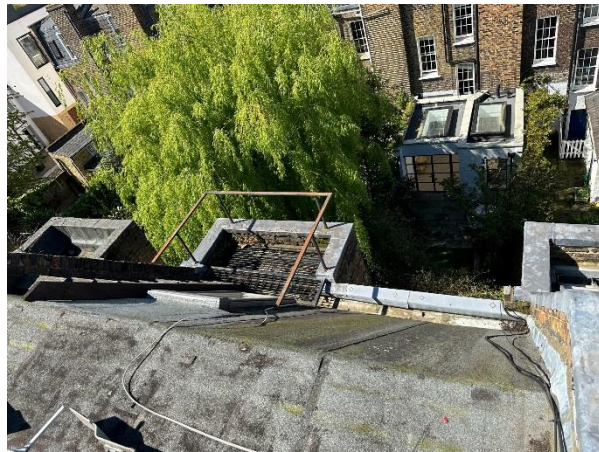
Fig 8. View showing No.17 rear roof
