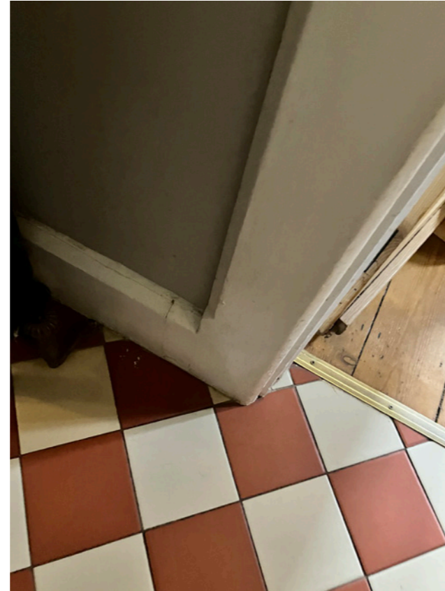
Non-original tiles internally
