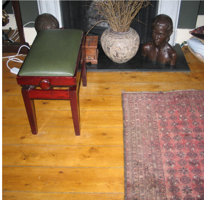
Floorboards to living room
