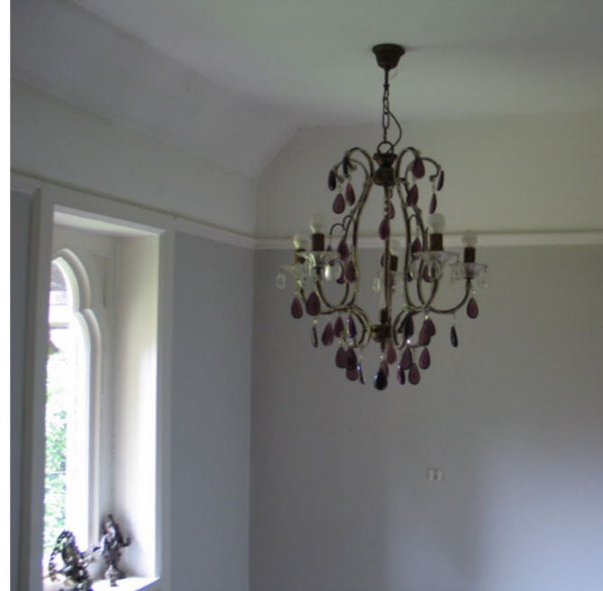
Existing chandelier to be removed
