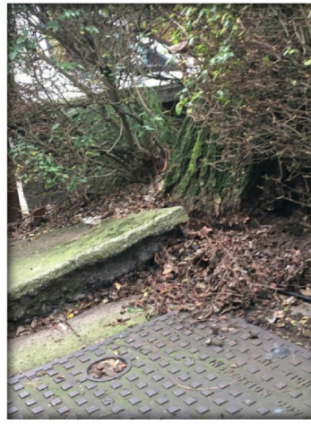
Image 6: Direct damage caused by tree to the private path in proximity to drain
