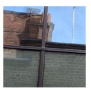
Our Corporate W20 range could be described as our "go to" product, it provides the advantage of narrow elegant profiles, offering the closest match to earlier steel framed windows and doors. The frames are hot dip galvanized for corrosion protection and factory powder coated to any RAL colour in our in house paint plant. The system can be both single glazed and double glazed as required with double glass offering centre pane u values of 1.1 which when assessed in line with EN14351
