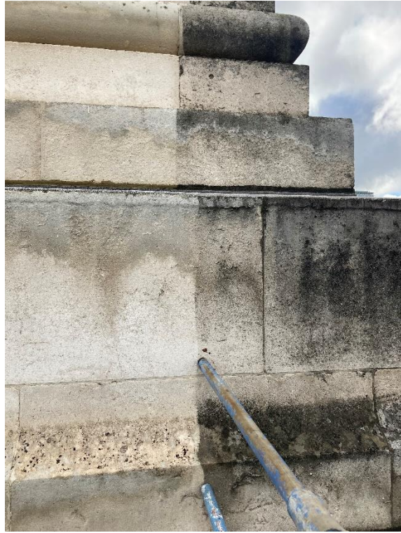
Stone cleaning to rear of tower, to right hand side
