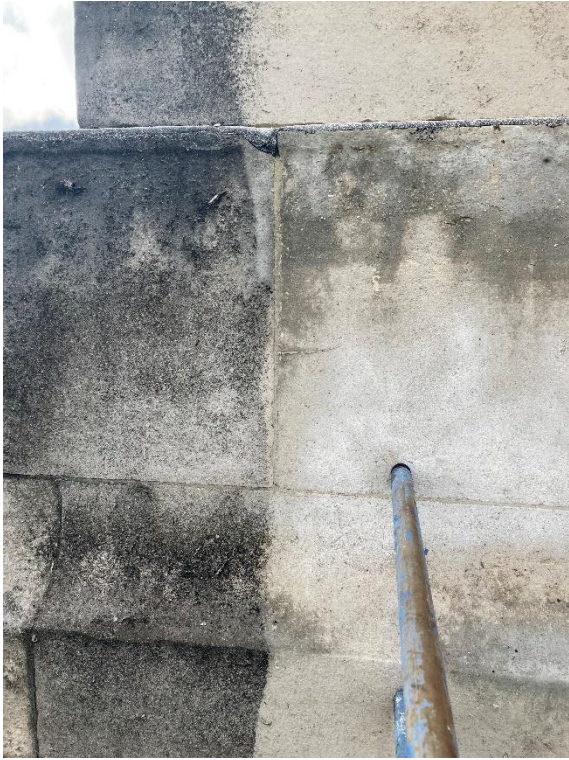
Stone cleaning to rear of tower, to left hand side
