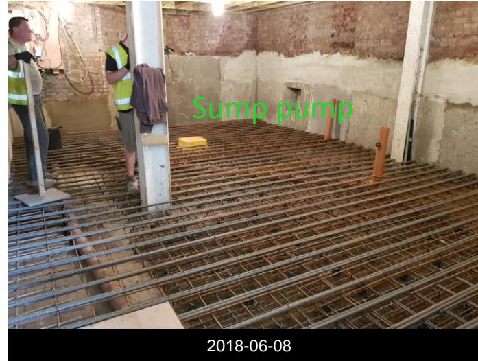
Steel work for cellar floor connected to wall pins
