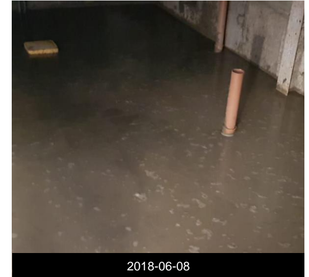
Concrete pouring for cellar floor: Completion of structural works
