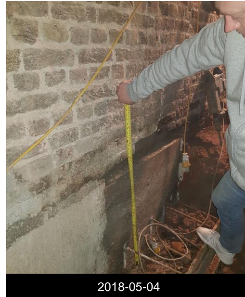
Detail of wall underpinning
