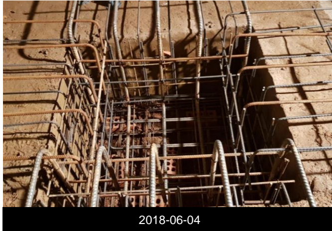
Sump pump chamber's steel work reinforcement
