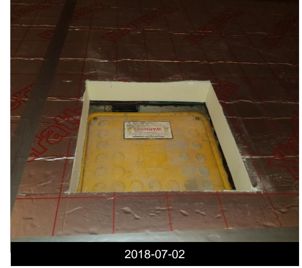
10cm Kingspan thermal insulation boards with access to sump pump chamber
