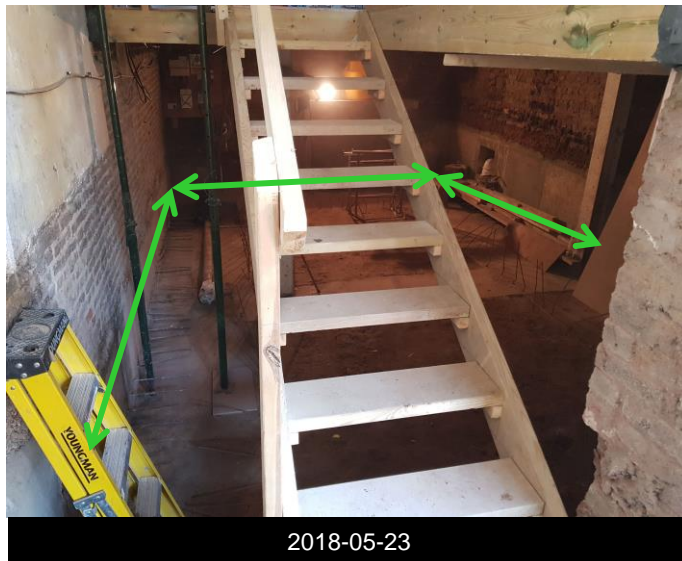
Walls and floor concrete underpinning complete
