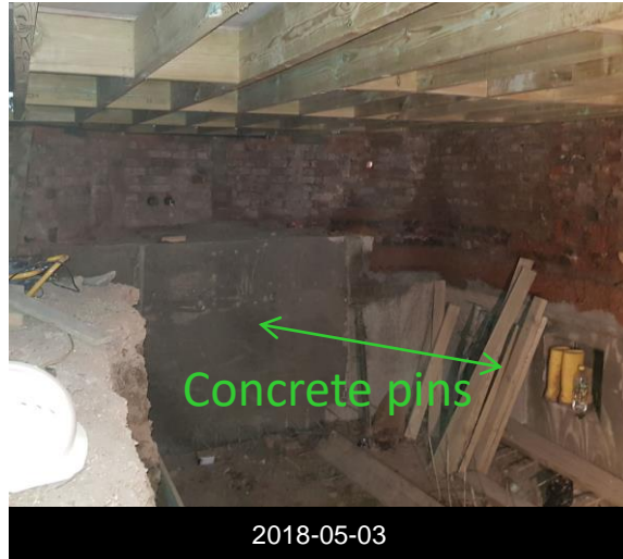
Concrete pins progression
