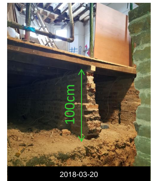
Cellar/Ground air gap
