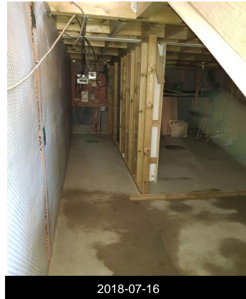
Erection of partitions
