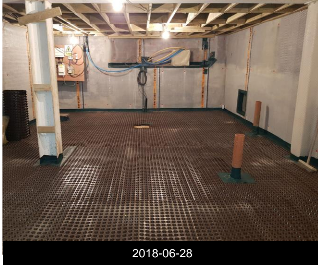
Insulation waterproof wall and floor membrane installation throughout
