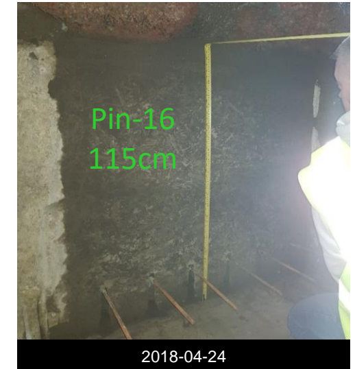
Detail of wall underpinning and steel ties connection to floor
