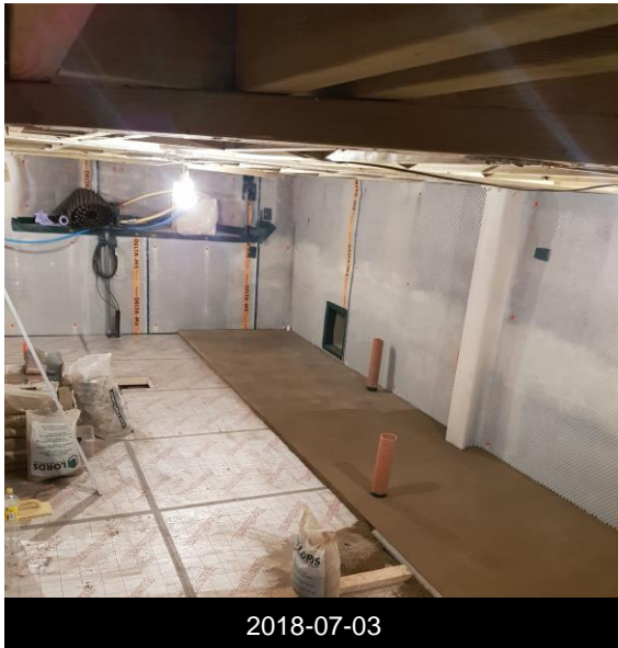
Layout of sacrificial 7cm floor screed covering the Kingspan insulation floor boards.
