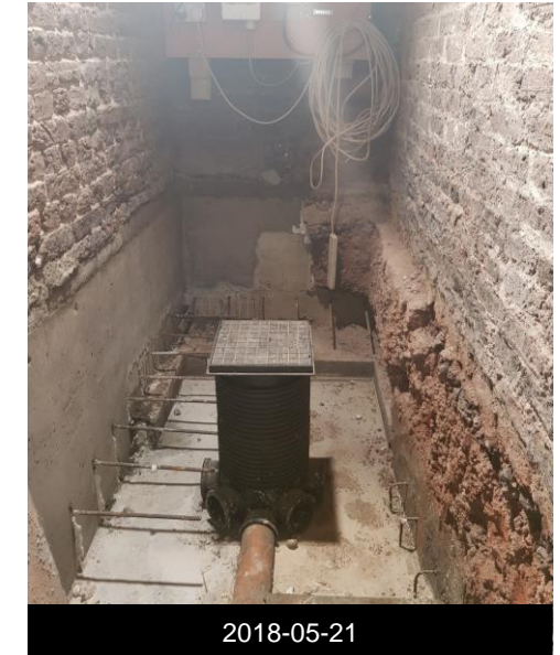
Sewage inspection chamber
