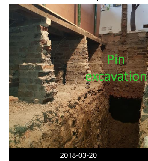
Excavation to accomodate concrete pins
