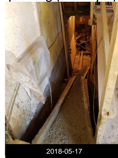
Floor concrete pouring (first layer)
