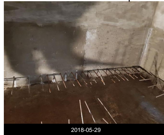
Detail of wall pins with steel ties connection with floor pins
