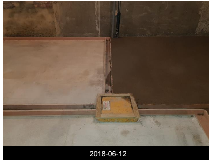
Floor channeling system from walls to sump pump
