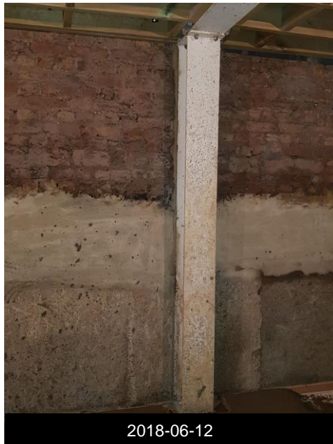
Detail of new cellar steel beam and column
