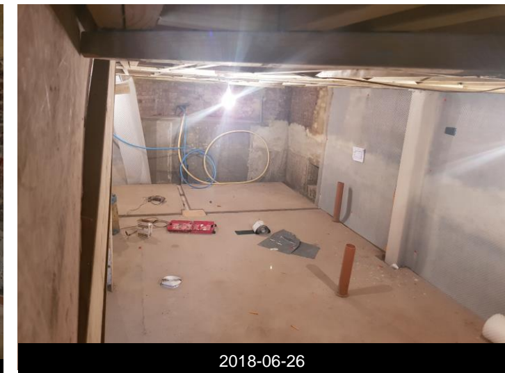
Floor screed and sump pump channelling details
