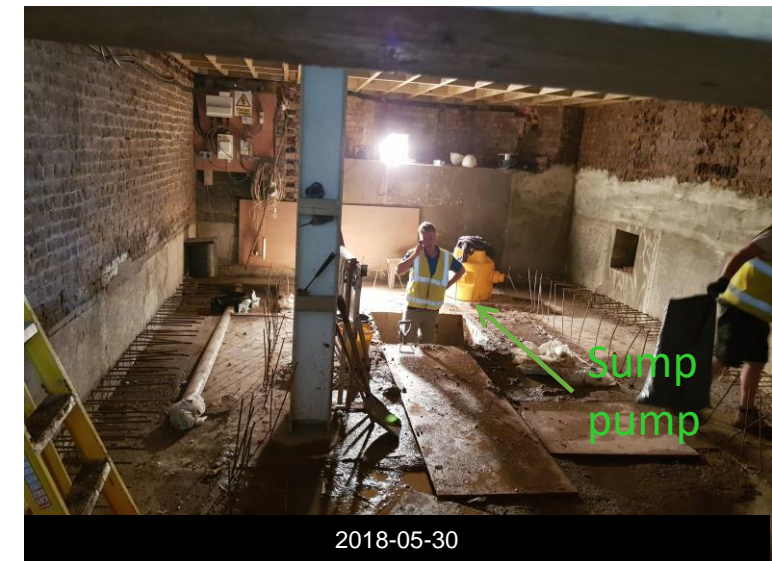
Floor steel work and sump pump chamber preparation
