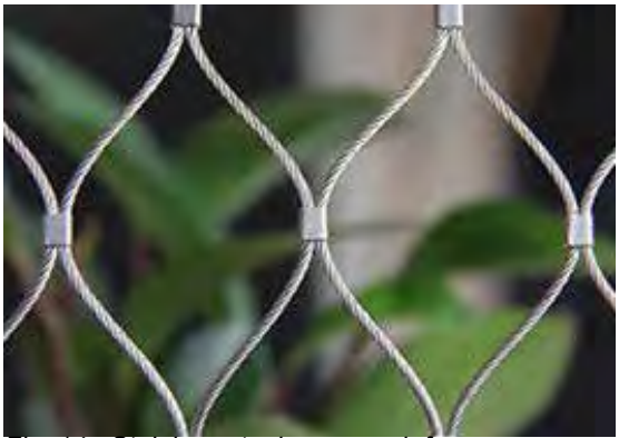
Fig. 14 - Stainless steel rope mesh for rear screening of roof terrace.
