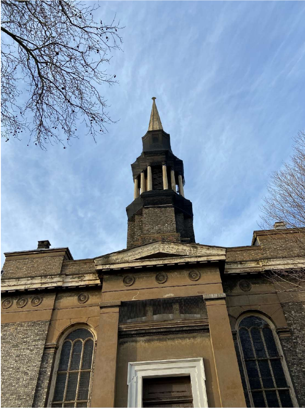
Img. 3; Black netting installed to tower
