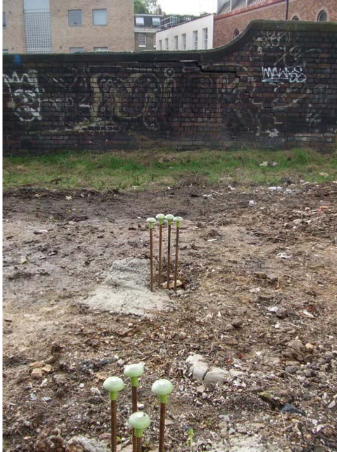
PHOTO 6: View southwest towards railway line, 17a Murray Mews and The Irish Centre with top of pile foundation and reinforcement bars seen in foreground.
