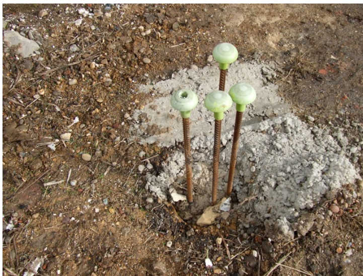
PHOTO 3. Close up of top pile foundation with reinforcement bars projecting out.
