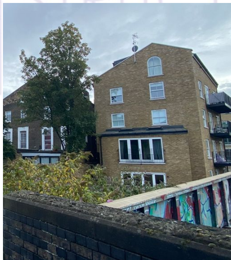
No. 3 St Augustine's Road rear view
