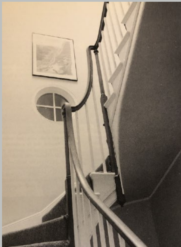
Plate 19. Wapping Pier Head 1813 - hardwood handrail
