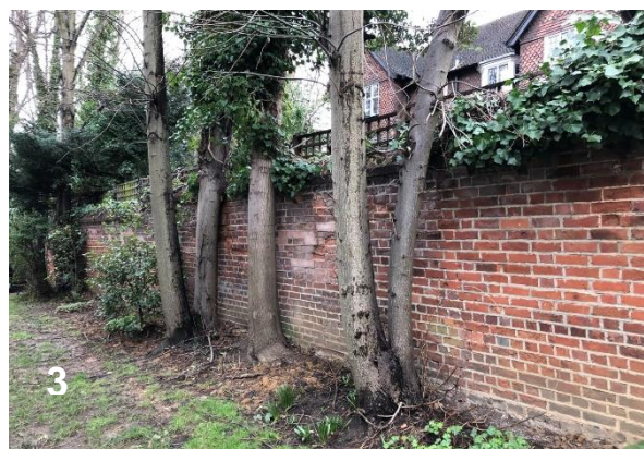
1. Image of existing dilapidated garden wall 2+3. Existing trees effectively supporting existing wall 4. Existing wall leaning towards neighbours garden
