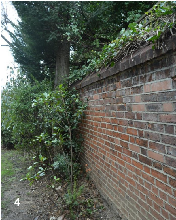
1. Image of existing dilapidated garden wall 2+3. Existing trees effectively supporting existing wall 4. Existing wall leaning towards neighbours garden
