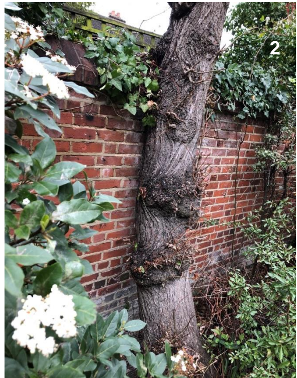
1. Image of existing dilapidated garden wall 2+3. Existing trees effectively supporting existing wall 4. Existing wall leaning towards neighbours garden
