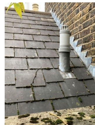
16 SVP venting to the rear pitched roof of no.6 Guilford Place
