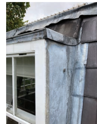
11 Leadwork detailing to dormer windows and mansard junction
