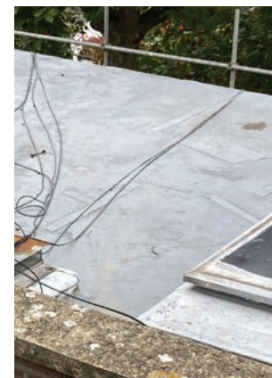
10 Patch repairs to flat roof membrane over no.3 Guilford Place
