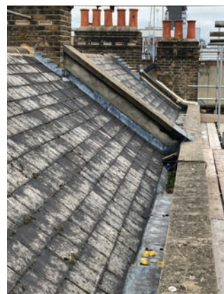
15 Synthetic slates to existing roofscape of no.5 Guilford Place
