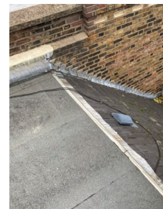
14 Felt covered crown roof to no.4 Guilford Place with brickwork party wall to no. 3 Guilford Place
