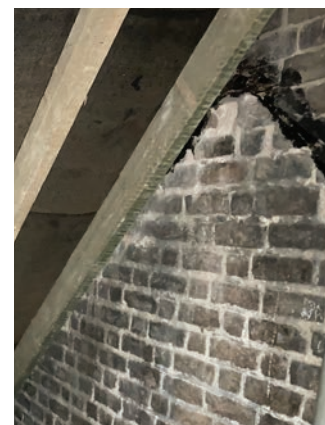
13 Brickwork markings of original roof pitch to no.4 Guilford Place prior to crown roof construction
