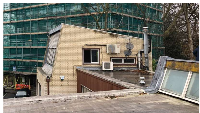
Fig. 6 Condensers fixed to Garage wall at high level
