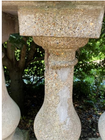
Figure 9 Fracturing/spalling of bottles
