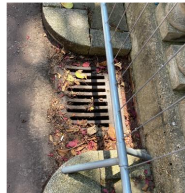
Figure 3 Drain grilles roadside of the balustrade plinths
