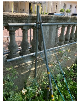
Figure 14 Scaffold buttress installed towards south end
