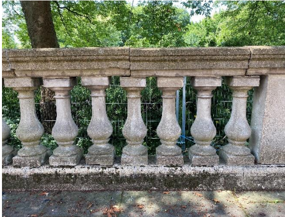
Figure 11 Differential coping levels
