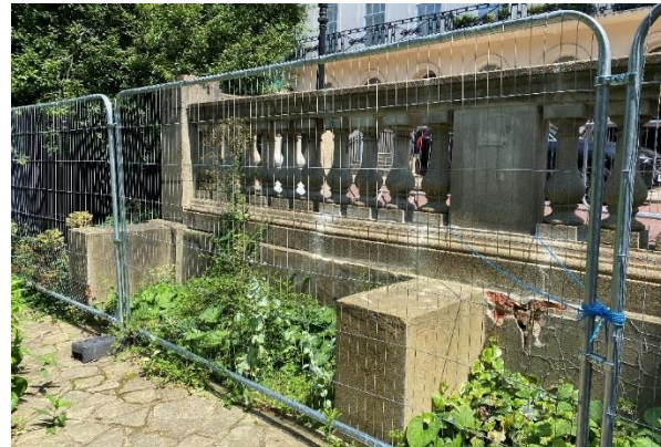
Figure 5 Balustrade as viewed from within the gardens. Note the kentledge blocks to resist lateral wall loading
