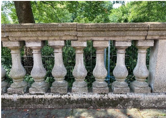
Figure 4 Balustrade as viewed from Chester Terrace. Note the step in coping level.
